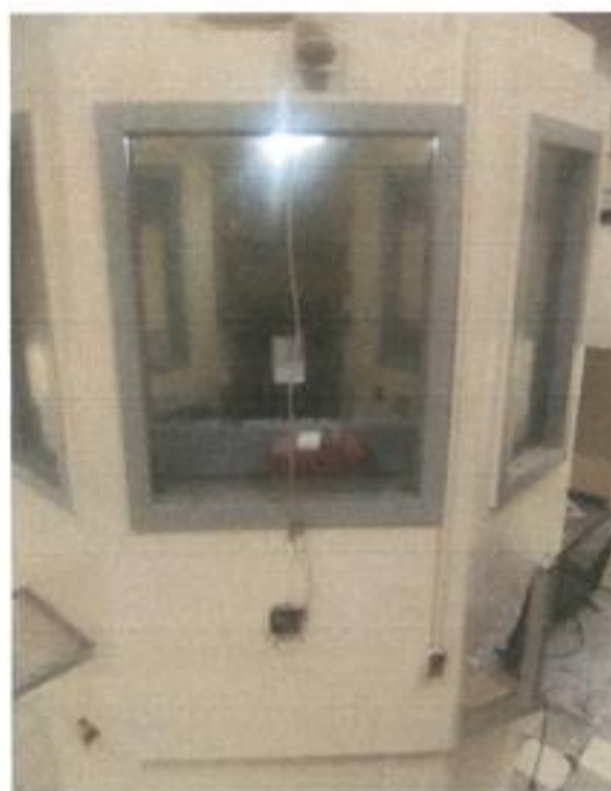
Parchman inmates say many prison towers, which once held correctional officers, now sit empty. This is an empty tower at Unit 29 "A" building. Mississippi Department of Health
